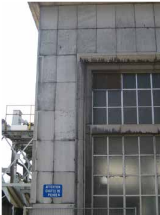
Viesville - Station de pompage
